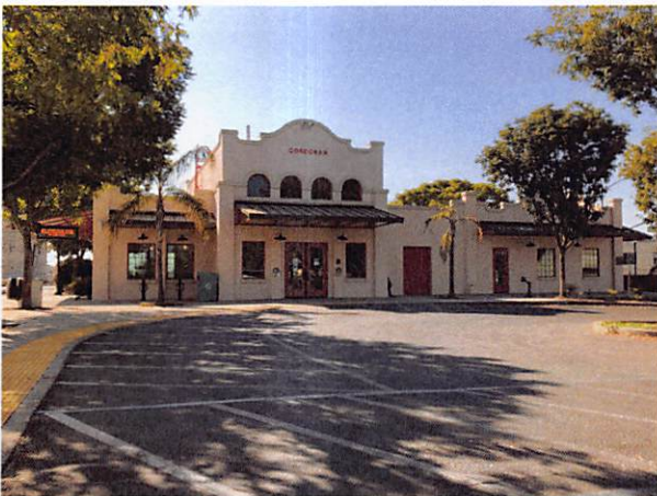
Corcoran Depot Building
