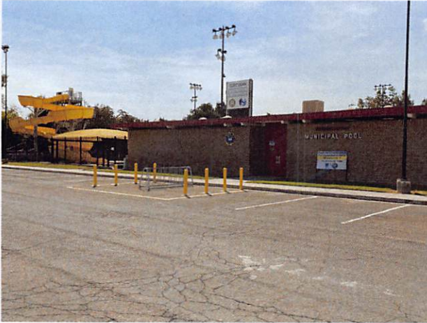
Corcoran Pool Building
