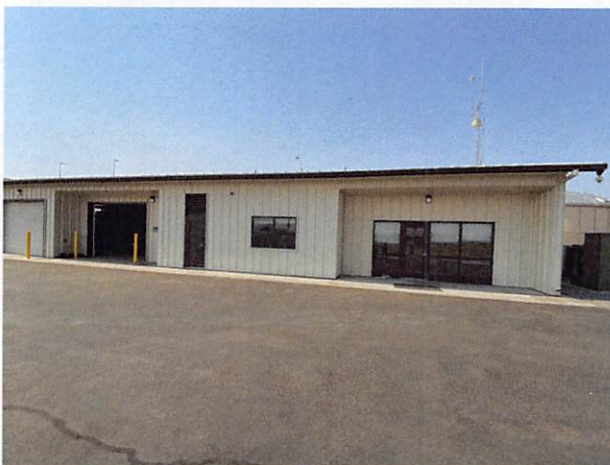
Corcoran Water Division Building
