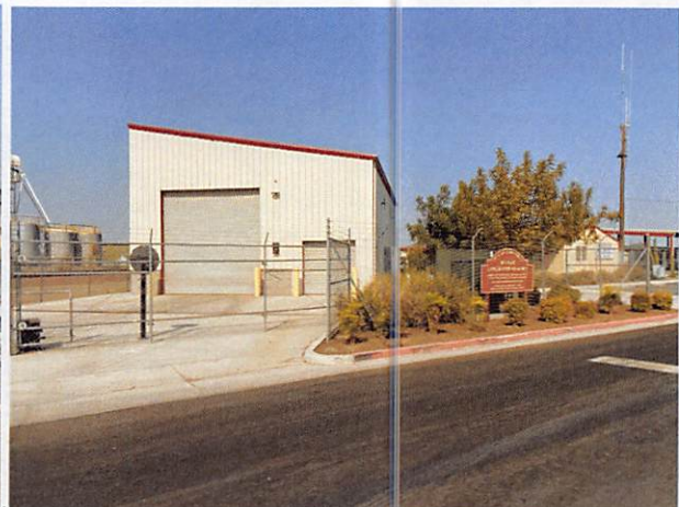
Corcoran Bus Wash Station Building
